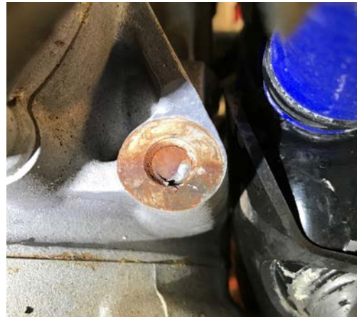
Fig.1 This picture shows the seized remains of a Europa/Rotax 912 engine mounting bolt: clearly this bolt had been broken for some considerable time and its failure led directly to a further bolt failure and extensive cracking of the engine mounting frame.
