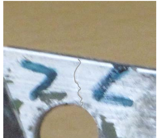
Fig. 1. Close-up of the Hub Bar crack
