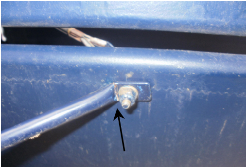
Figure 2: View from underneath horizontal stabiliser showing crack at flattened end of strut.
