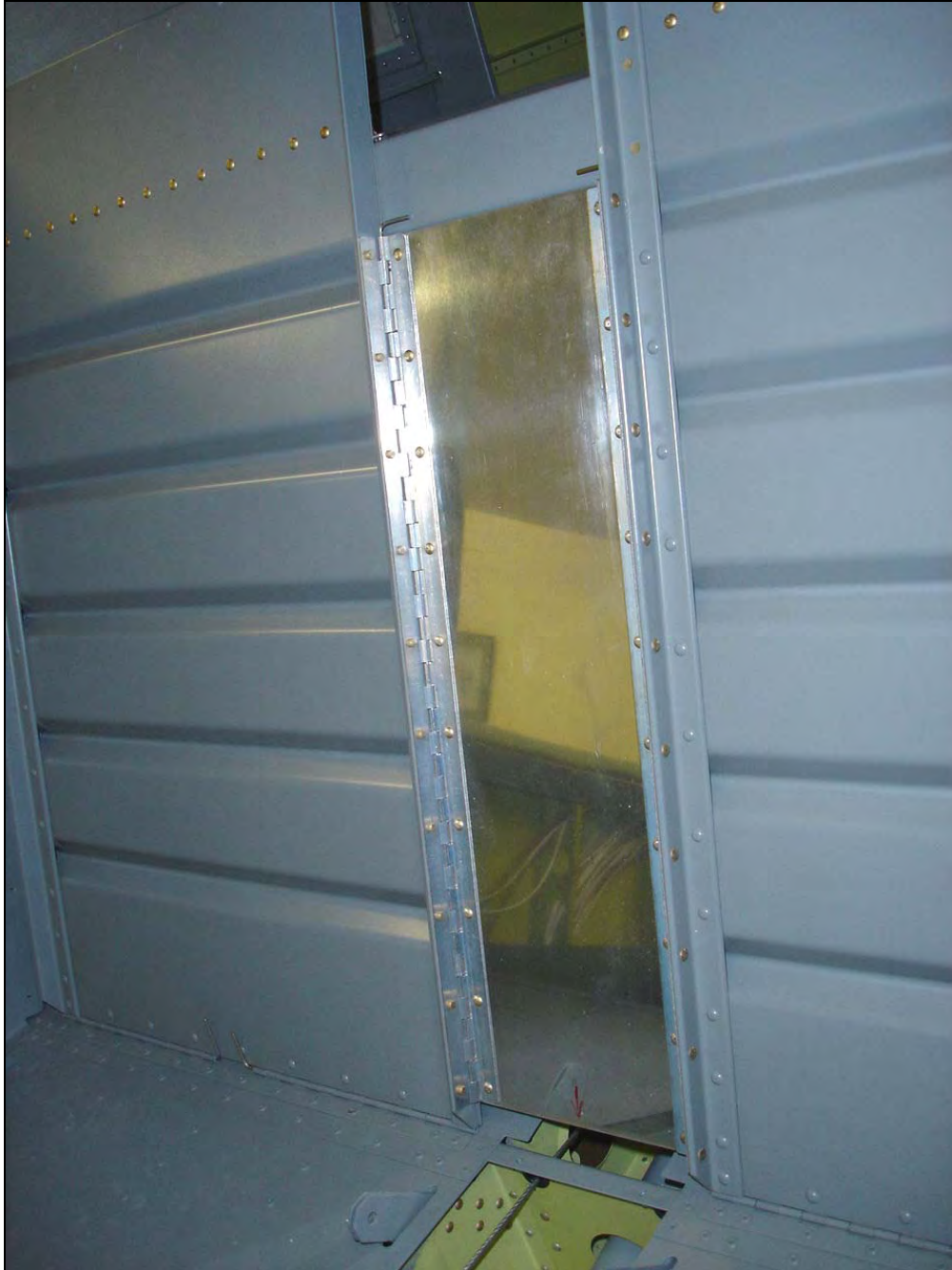
Picture 3 Finished assembly, view looking aft
